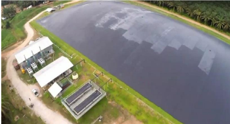
Figure 7.12: Installation of liquid palm oil waste processing plant with biogas technology to produce bioelectricity in East Kalimantan province
