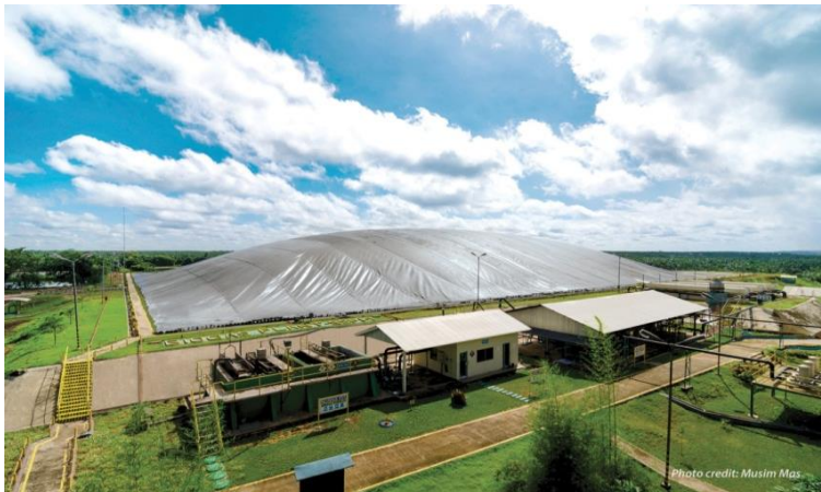
Figure 9.3: Biogas-generated Power Plant/Methane Capture (Bioelectricity) at the Palm Oil Mill Waste Management Facility in Riau Province.
